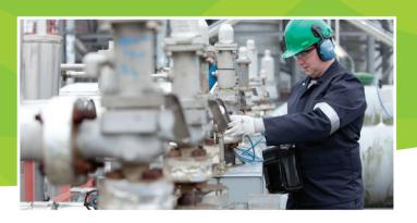
Fugitive emission management (LDAR) (Leak Detection and Repair)
